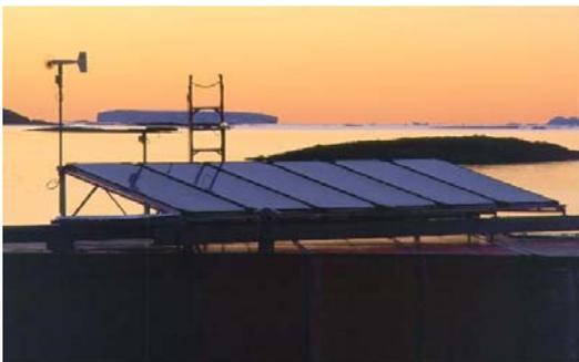
The Non Residential Systems are large, “active”, “closed circuit” systems to cater for hot water demands in excess of 2,500 litres per day. These systems use a “drain back” principle and hence the collectors must be installed at a higher level than the heat store. The ‘M’ or ‘B’ collectors and the “drain back” principle make these systems suitable for any situation:
